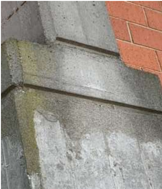
Image 6: Humidity due to weathering
