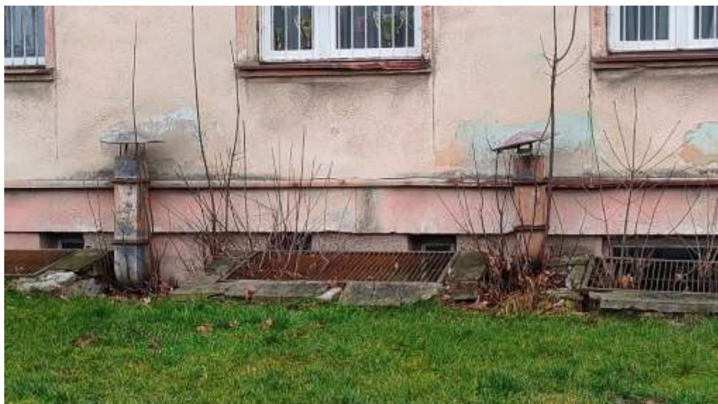
Photo 15. The ventilation system is outdated and requires audit and replacement.
