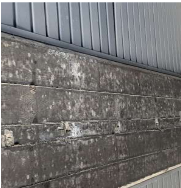
Image5: Moisture attacks load-bearing structures, creating thermal bridges where there is a change of material/structure, leading to hygrometric consequences in flats
