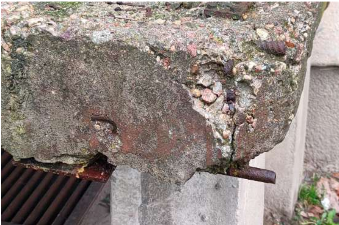
Photo 5. Entrance platform showing detachments as well as exposed and rusted reinforcement iron.
