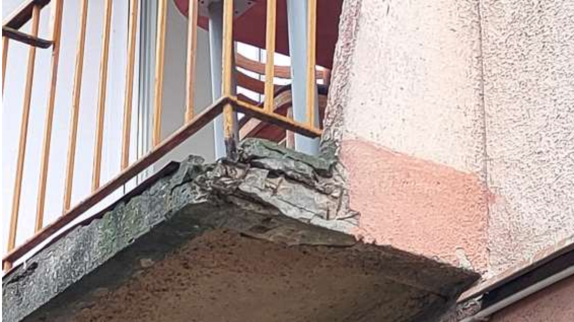
Photo 6. Balconies showing cracks and detachments as well as exposed and rusted reinforcement iron.
