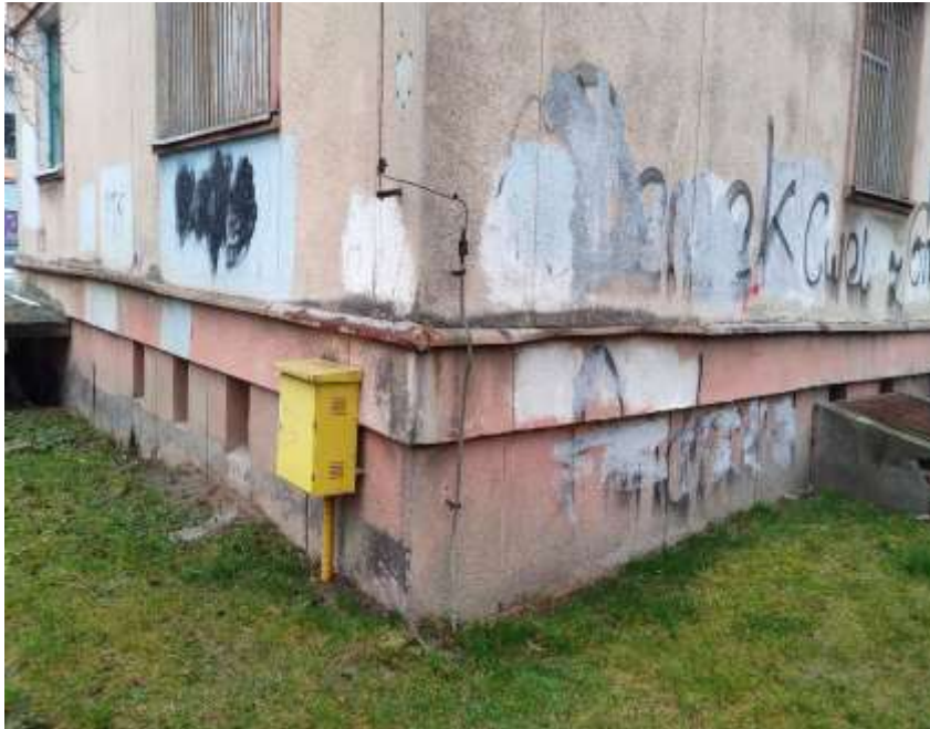
Photo 8. Lack of exterior insulation and damages to sheet metal flashings, resulting in humidity issues inside and outside of the Building
