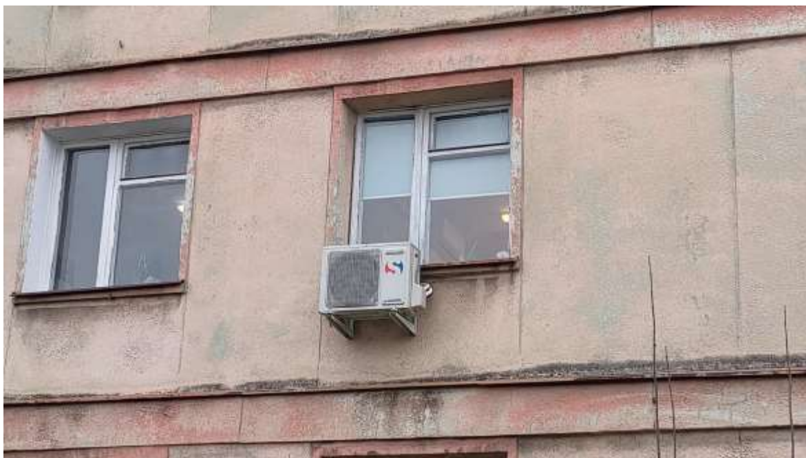
Photo 2. Individual air condition device (split type).
