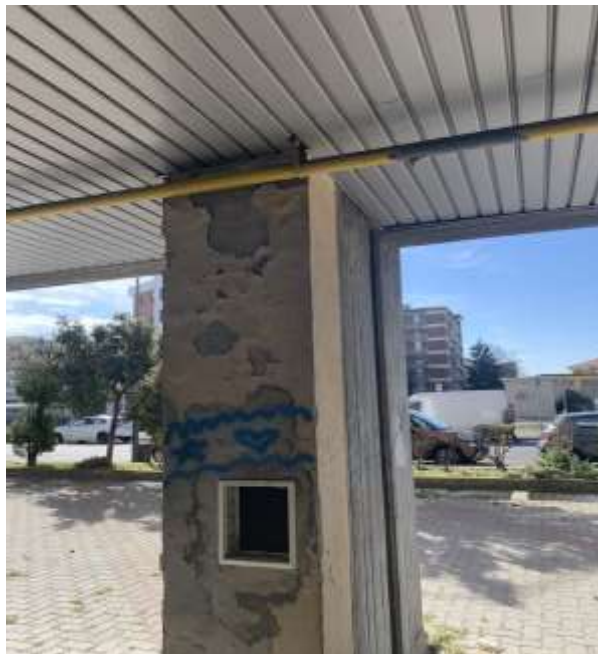
Image2: Technological cavity accommodation masonry showing the state of deterioration of the masonry
