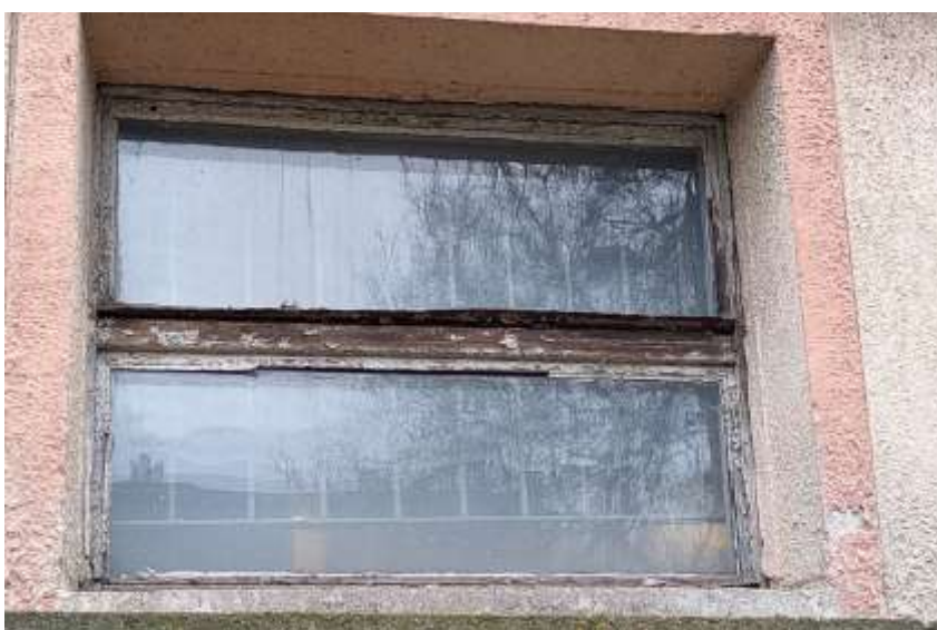
Photo 9. An old window in extremely poor condition, with peeling paint and damages to metal flashings, all due to the lack of regular and proper maintenance
