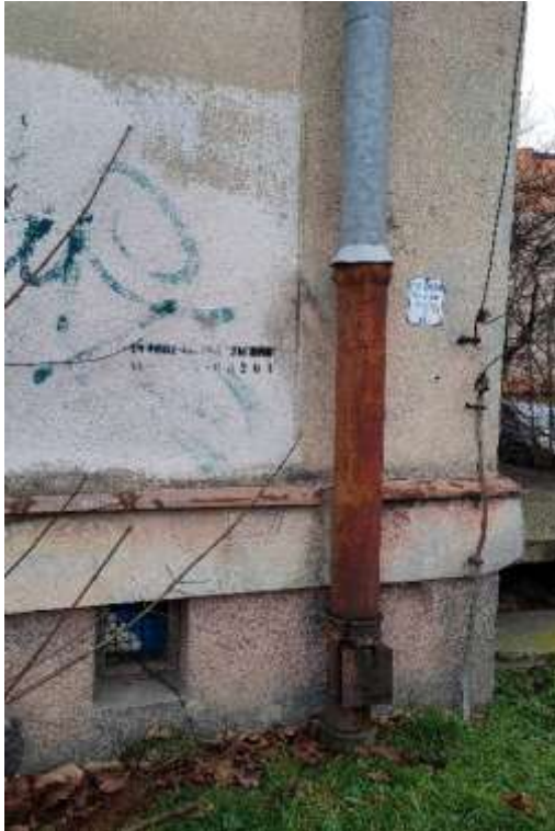
Photos 10-11. Damage to a drain pipe due to frost or mechanical force, resulting in the increased water penetration of the foundation walls and in turn – increased humidity.
