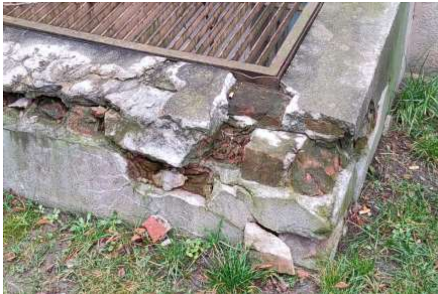
Photo 3. Degradation of basement windows structure due to water infiltration and mechanical force
