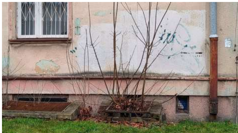
Photo 13. Self-seeded trees and bushes destroying brick basement windows structures and allowing for water penetration into the walls.
