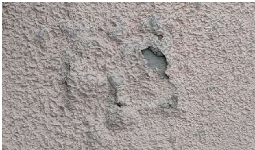
Photo 4. Exterior walls showing the state of deterioration of the plaster due to thin layer and humidity
