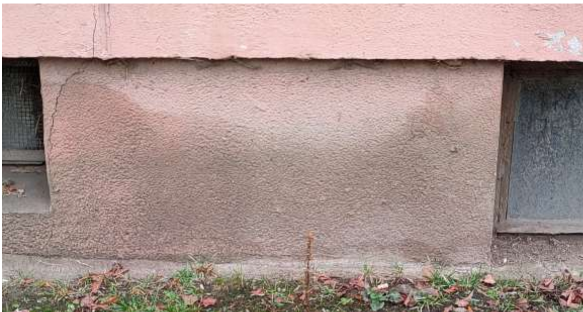
Photo 7. The concrete foundation wall shows visible signs of rising humidity presence
