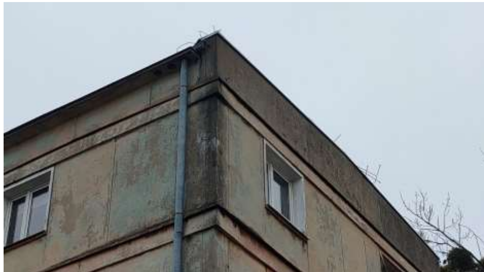
Photo 12. Humidity due to weather and damages to roof flashings.
