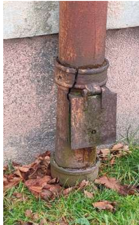
Photos 10-11. Damage to a drain pipe due to frost or mechanical force, resulting in the increased water penetration of the foundation walls and in turn – increased humidity.
