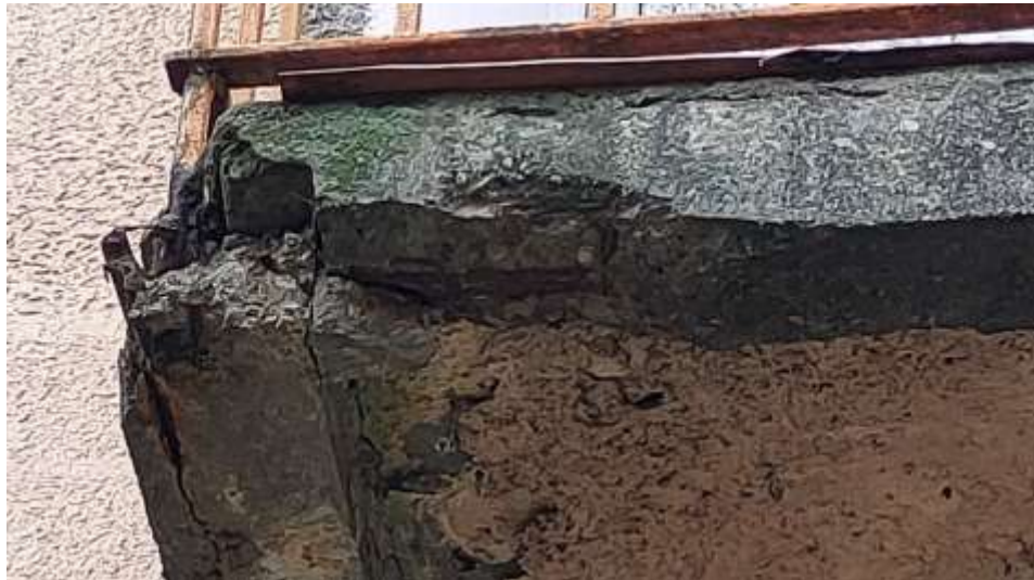
Photo 14. The balcony shows evidence of concrete detachments due to wear and tear and damaged metal flashings, mostly subjected to water infiltration; gravel nests due to the inadequate mixture.
